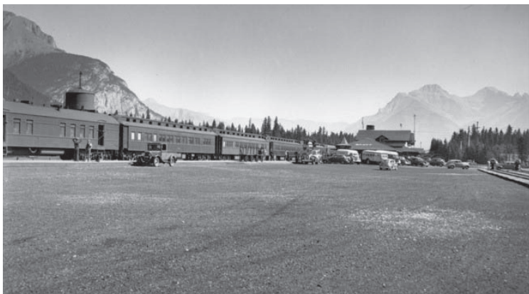
FIGURE 4.05 Historic view east to the station
