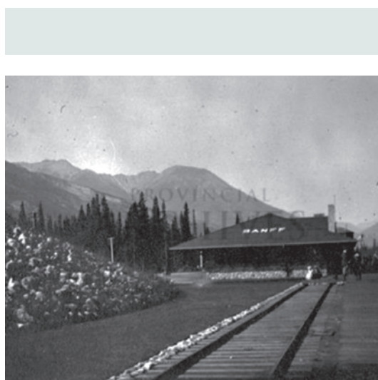
FIGURE 7.10 CPR garden with single 'green track', potentially prior to the addition of the Spruce Allée.
