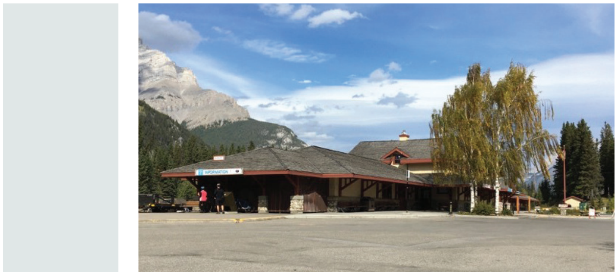
FIGURE 4.17 West end of Banff CPR Station
