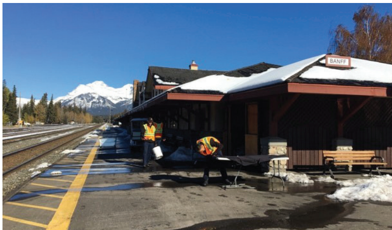
FIGURE 4.03 Looking east along platform of the Banff Canadian Pacific Railway station
