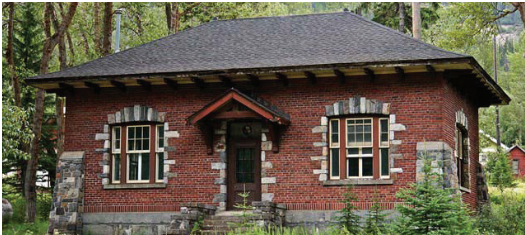
FIGURE 7.16 Field Telegraph Building
