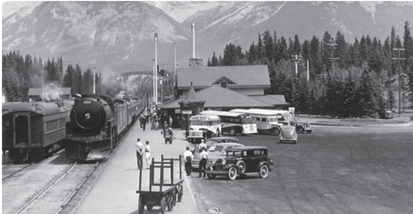
FIGURE 1.02 Westbound passenger train arriving into Banff Station
