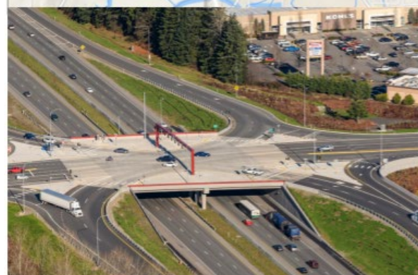
Aerial view of the completed 116th Street NE interchange looking northeast.
